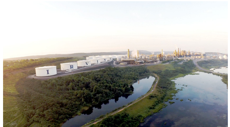
Irving Oil Refinery, Saint John, N.B.
